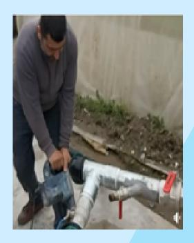
Two multi-sensors were installed in the Tarsus (TAR) pilot site, located in southeastern Turkey, at the eastern coasts of the Mediterranean. The two sensors record in real-time critical parameters related to salinization, such as electrical conductivity (EC), pH, Eh, dissolved oxygen and, water level.
