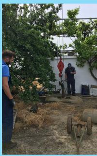
Three (3) more sensors have also been installed at the Rhodope (RHO) pilot site in Eastern Greece. The installation required the modification of boreholes to accommodate the multi-parameter sensor in a separate and safe tube and includes full energy supply and remote data transmission.
